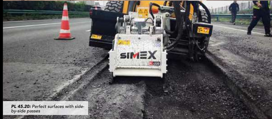
PL 45.20 HP: Resurfacing road failure.
