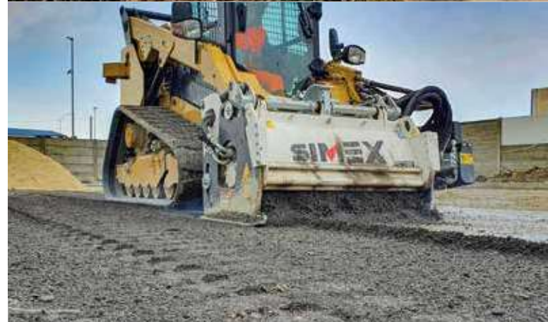
PL 1000. Resurfacing industrial yard.
