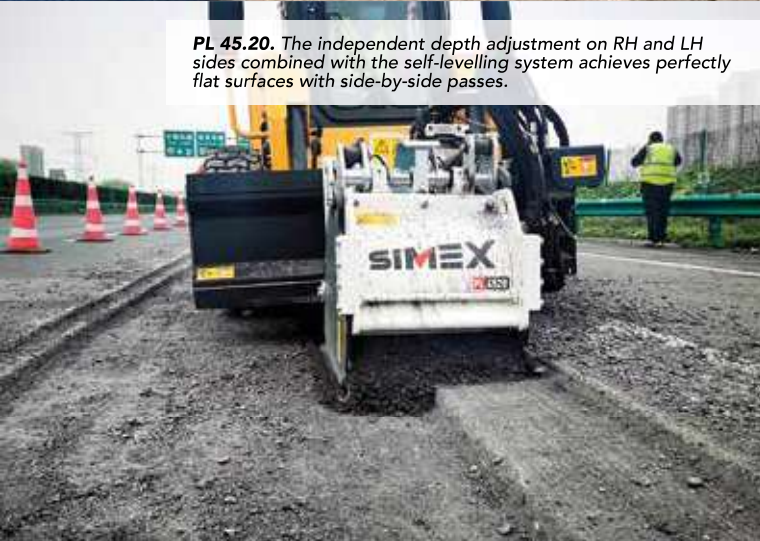
Detail of milling depth during road repair work.
