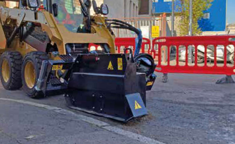
T 300. Construction of micro-trench with 25 mm wide disk.
